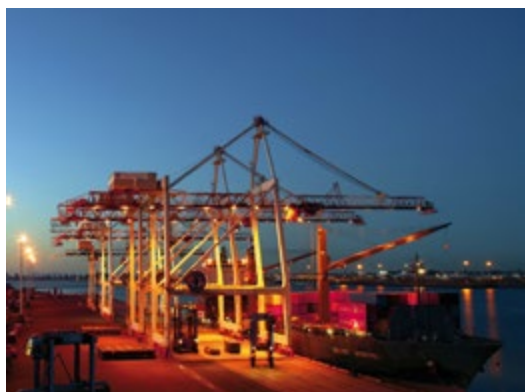
Ship to shore cranes.
