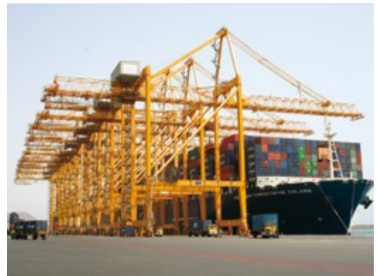
Ship to shore cranes.
