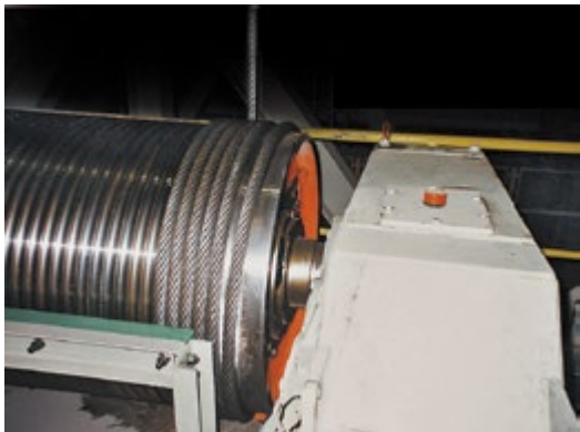
Hoisting mechanism in a steel picking line.
