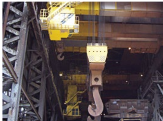
Travelling crane in steel mill.
